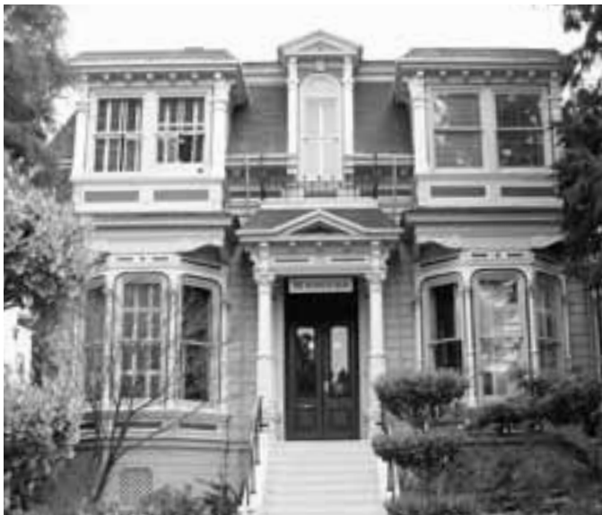
Edward Childs built this home in 1880 for Adolph Schnabel. Childs' design combines elements of the Italianate style with the Second Empire style's mansard roof. The home is now an office building called "The Mansard Building."
