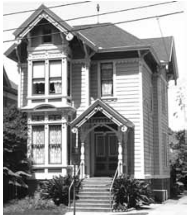
Robert Harvey built his Park Avenue home in the "modern" style adding square windows, rather than the bay windows inherent in the Italianate style. He also dressed the home with geometric ornaments and anticipated the Queen Anne-style with fish-scale shingles. Today we call Harvey's "modern" style "Stick" or "Eastlake."
